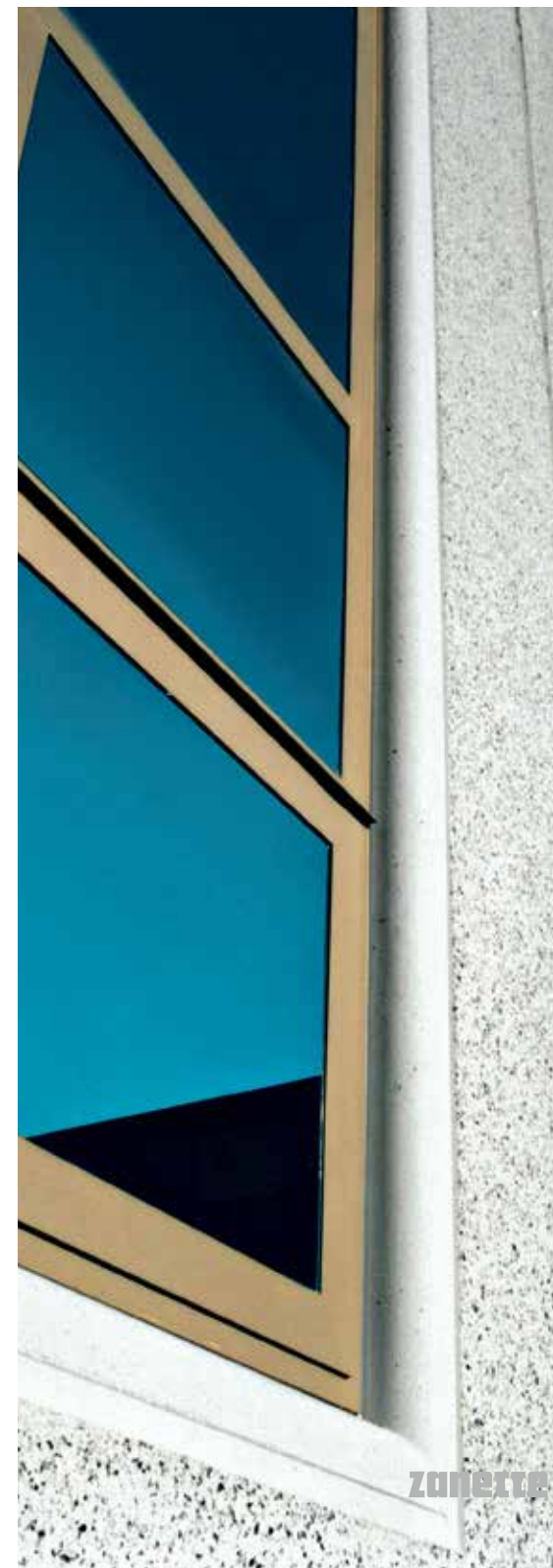
| Detail of windows mouldings
